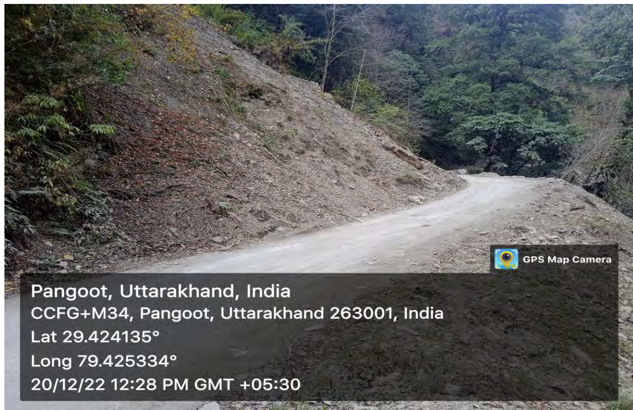
Landslides resulting due to exposure of roots in the process of vertical hill cutting.
